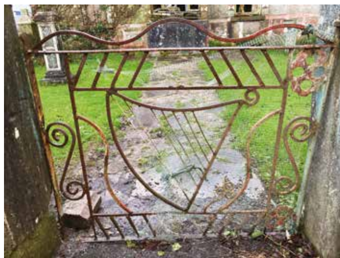
Wrought iron Celtic revival motif used in a pedestrian domestic gate outside Lixnaw.
