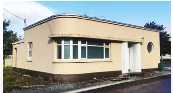
Gate lodge at Listowel District & Fever Hospital (1933–41) — John J. Winters. Credit: Author's own photograph.
