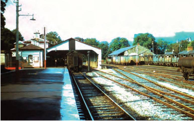
Plate 9: Killarney station on 15 September 1960 with a gas wagon on the right with two horizontal cylinders of gas for the Radion Train dining cars. Behind is a long train of cattle wagons as nationally cattle fairs were large in September and October with farmers downsizing their herds to conserve winter feed. (Source: Roy Denison)
