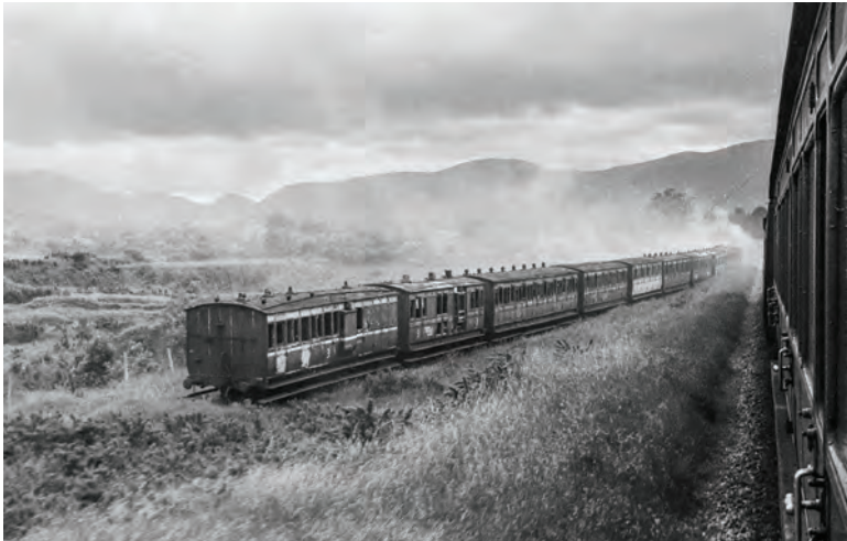
Plate 4: For the construction of the railway from Killarney to Tralee, the railway opened a large ballast pit on the North side of the railway from the back of Fair Hill, Killarney, to the Tralee Road overbridge. Overhead bins were erected on large wooden frames and wagons were shunted underneath and quickly filled. Large quantities of stone and gravel were extracted until the 1930s. The sidings were then retained for storing trains on busy GAA days. In 1957, old carriages that had been used in Cork for Summer Sunday excursions to seaside stations in West Cork were parked there and left to decay as seen on 10 June 1958. (Source: Roy Denison).
