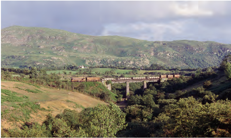
Plate 2: The Quagmire Viaduct in a scenic setting between Headford Junction and Killarney on 19 July 1985 with the 18:25 Freight train from Tralee to Mallow (Source: Barry Carse).
